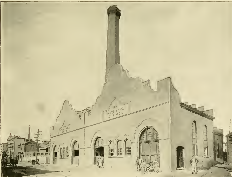
POWER HOUSE NEW JERSEY TRACTION CO., BOYD STREET.
